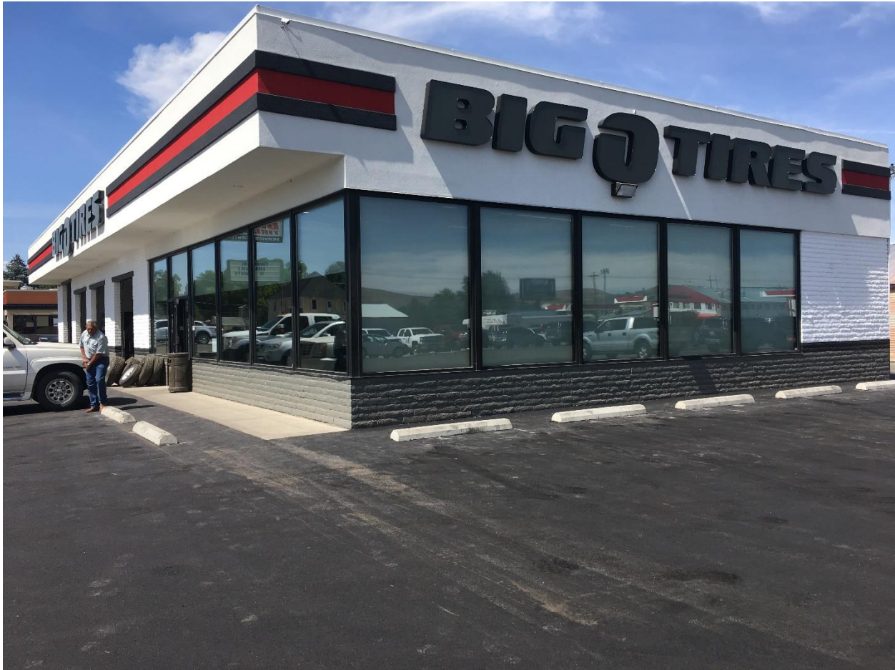
Current Store AFTER Renovation and Upgrades
