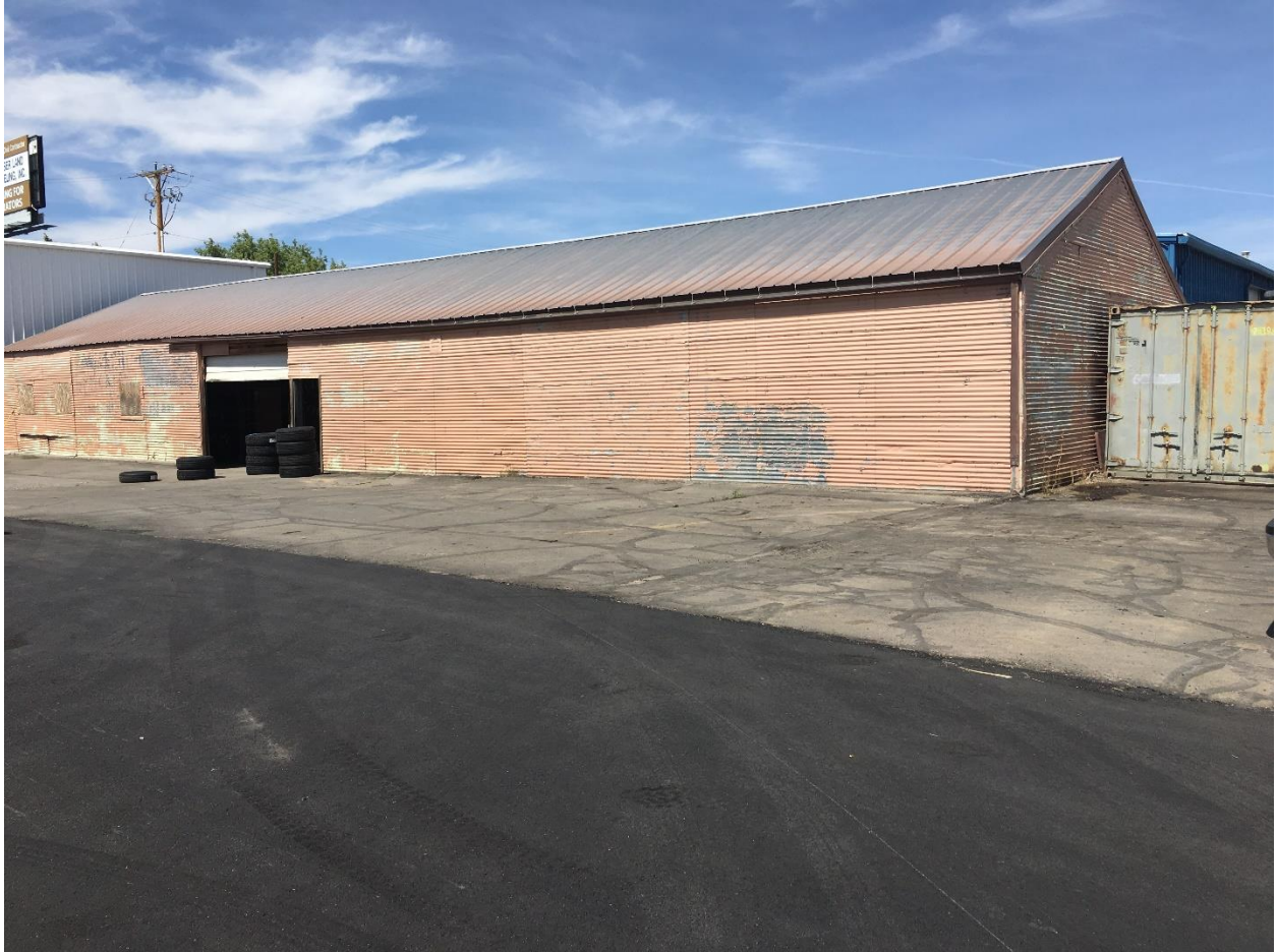
This Current Tire Storage will be demolished and the area paved
